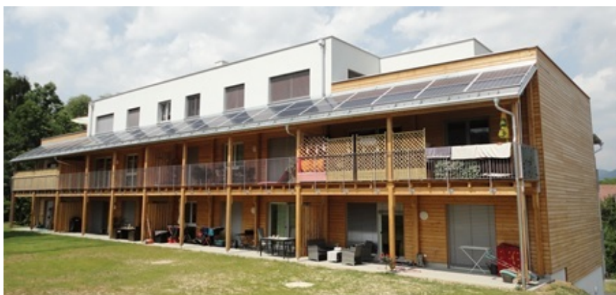
Figure 1-1 Building in Weiz (Hutter, 2016)
